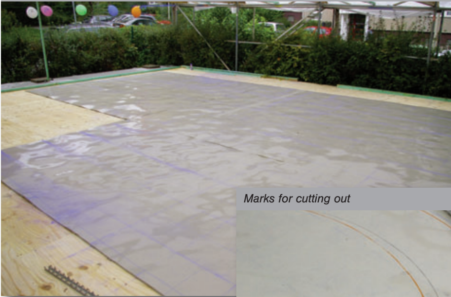
Formliners laid out onto formwork ground
