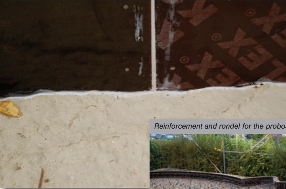
Sealing between formliner and frame
